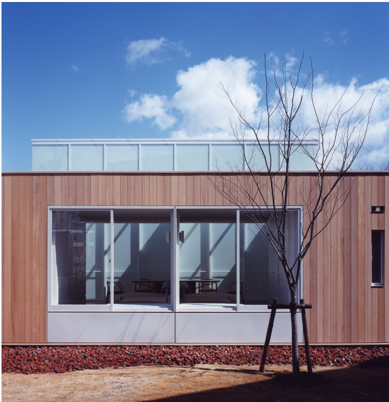
南西側宿泊室外観 view toward guest room from southwest
