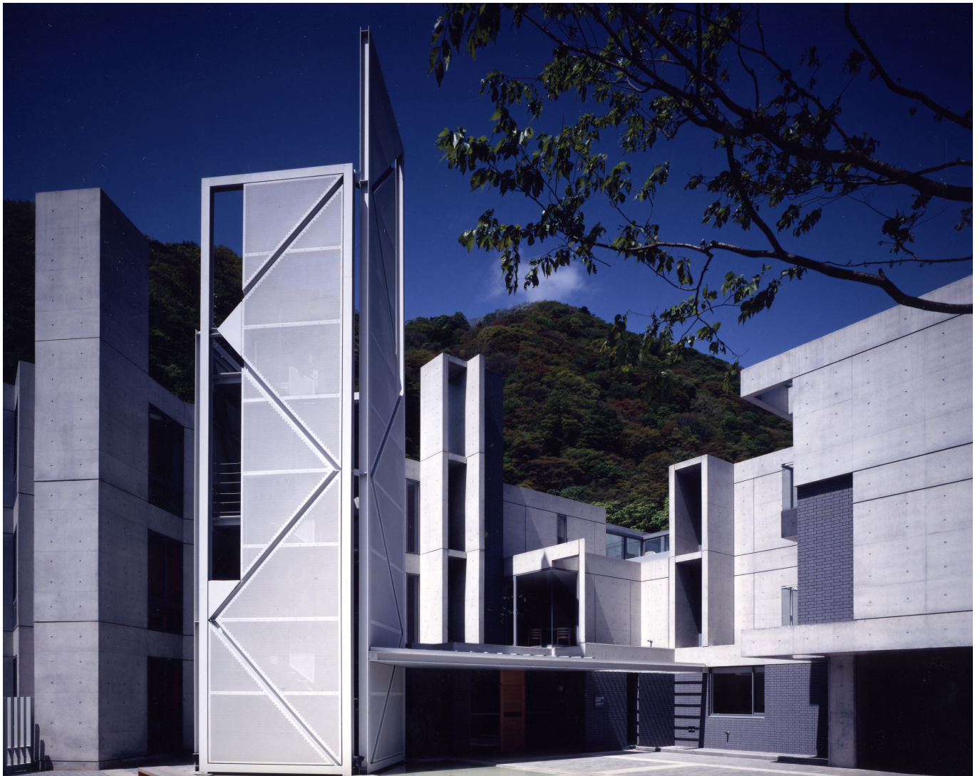
寮・東側外観 view from east
