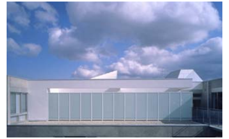
東側外観 view from east
